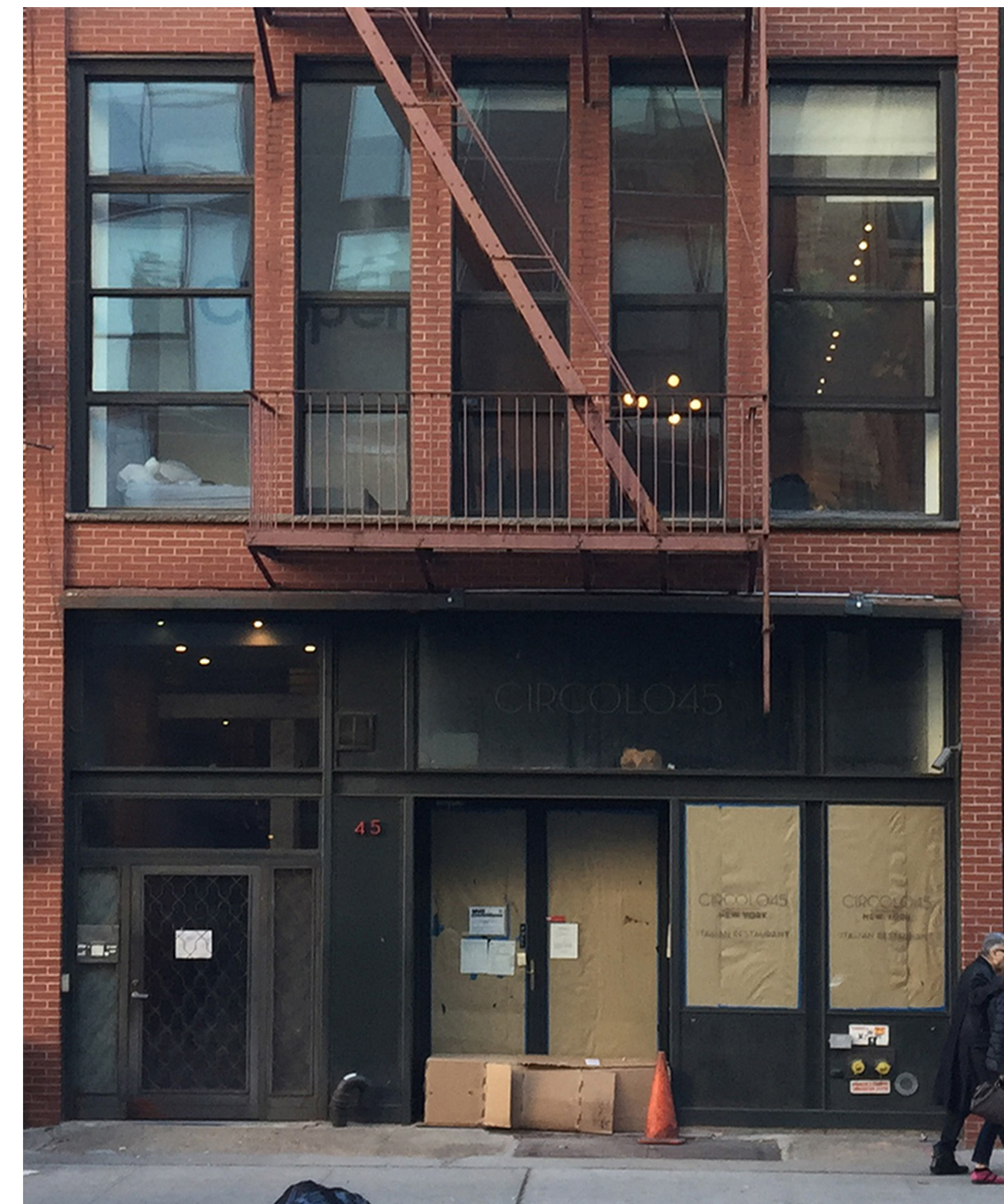
AREA OF WORK - EXISTING STORE FRONT
